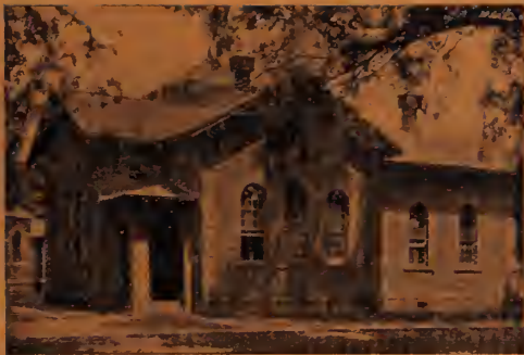
Sept. 6, 1896. "The old chapel built in 1847, which was characterized by Dr. Atwater as an 'architectural gem', is already razed to the ground."
